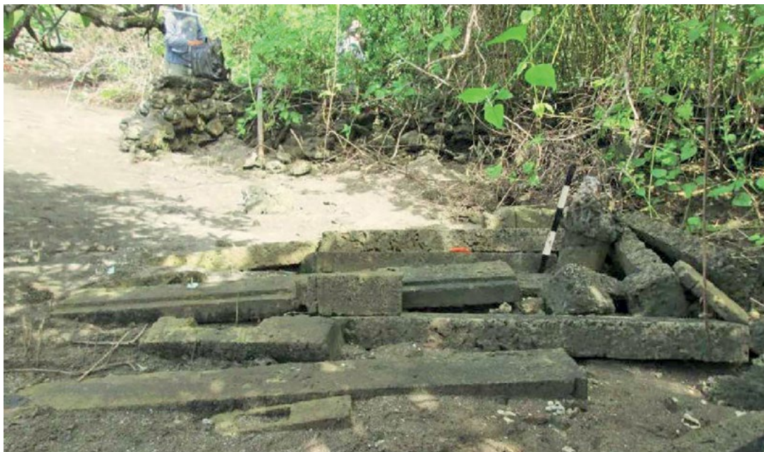
Figure 20.9: The Tosalama of Labuang's grave in deteriorated condition from beach spray abrasion.
