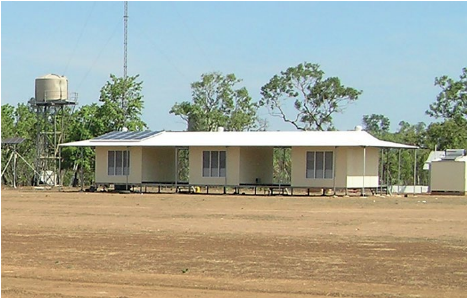
Figure 16.3 The three rooms in the single-man's quarters, constructed by volunteers and community members in 2008. Philanthropic funds donated through the Rotary Club of Melbourne financed the project.
